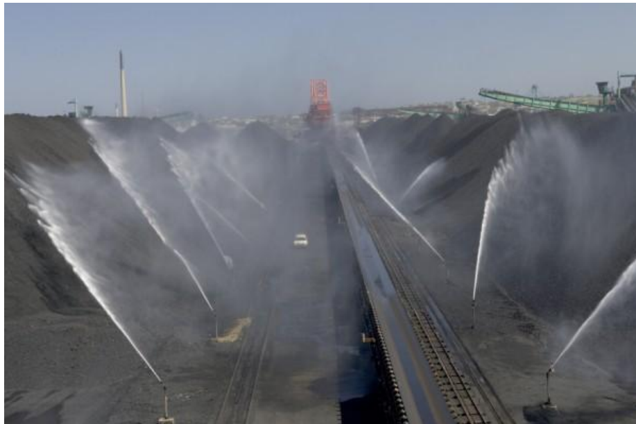
Numerous water sprays are located within the PKCT site. These retain high levels of moisture within the coal to limit the movement and escape of dust.
