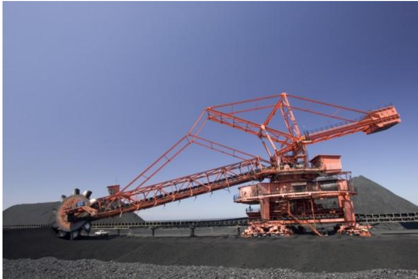
The bucket wheel can be moved laterally and vertically in order to fully collect coal. The operator is housed in a cabin just behind the wheel for optimum visibility. The bucket wheel deposits coal on a conveyor belt which transports coal to the ship loader. The white vehicle behind the wheel gives an idea of scale.
