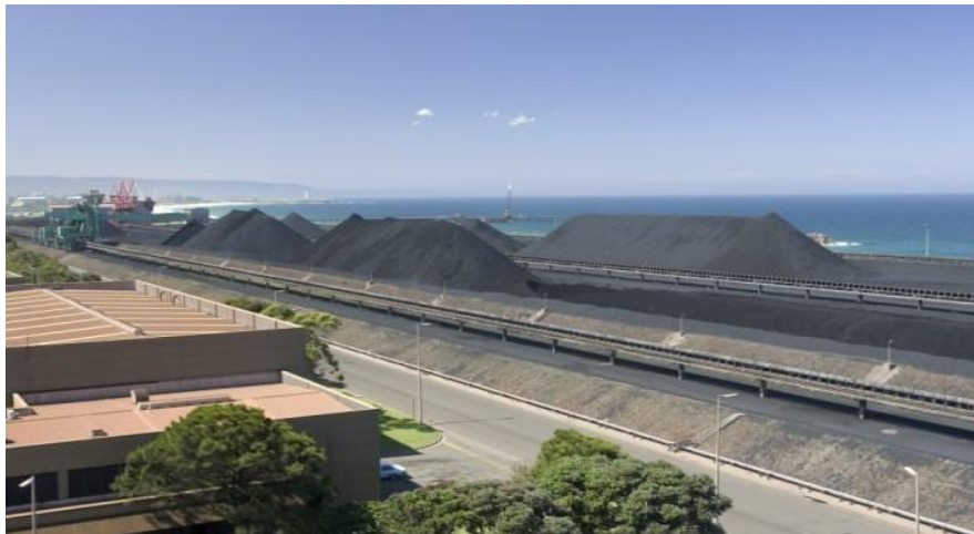
The stockpiles are located between the stackers with the bucket wheel reclaimers in-between the piles.
