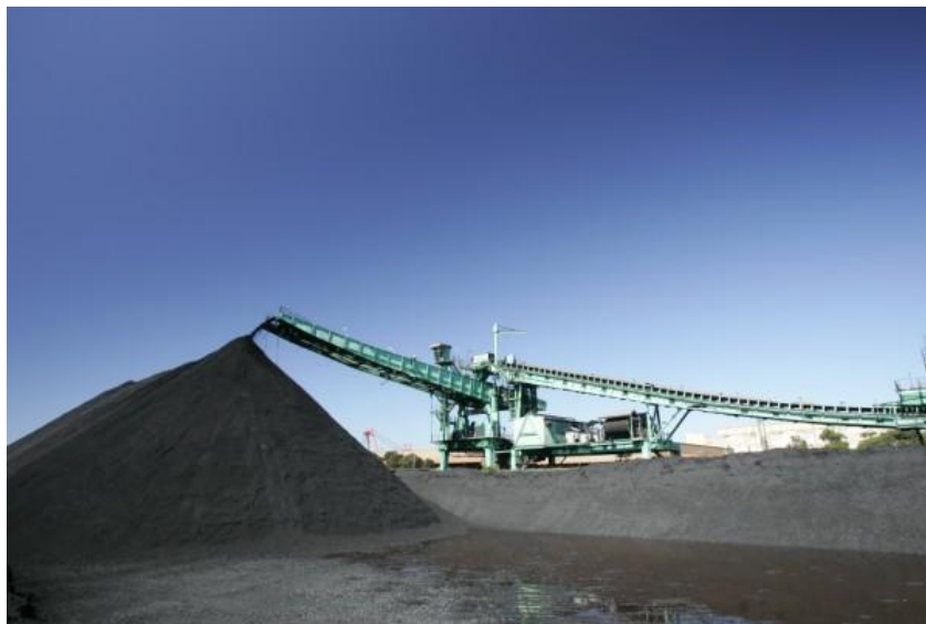
The moveable stacker deposits coal in organised piles depending on owner and type. PKCT has three stackers which operate effectively to accommodate high delivery levels. The stacker arm moves up and down to minimise coal dust movement by reducing the height from which coal is dropped.
