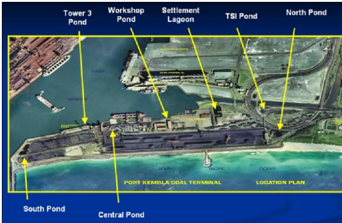
Figure 33 – PKCT Surface Water Infrastructure
