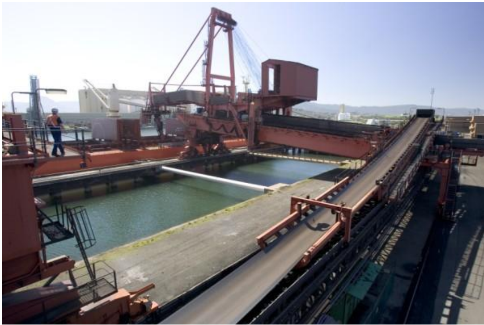
Coal from the bucket wheel reclaimer travels along the conveyor belt and in to the ship loader. The 'nose' of the loader drops into the hold of the ship to ensure minimum dust emissions. The loader moves laterally to access the different holds.
