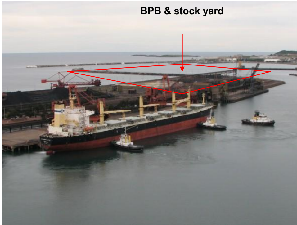
Materials are stored in the BPB stock yard prior to being loaded onto a vessel berthed at the number 101 berth.
