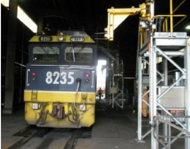
The coal delivery train unloads within a partially enclosed building to assist dust control.
