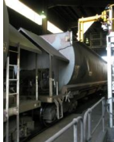
Coal is dropped from the wagon into a hopper for transportation to the stockpiles. Dust escape is minimised due to the enclosure of the rail reveal area.
