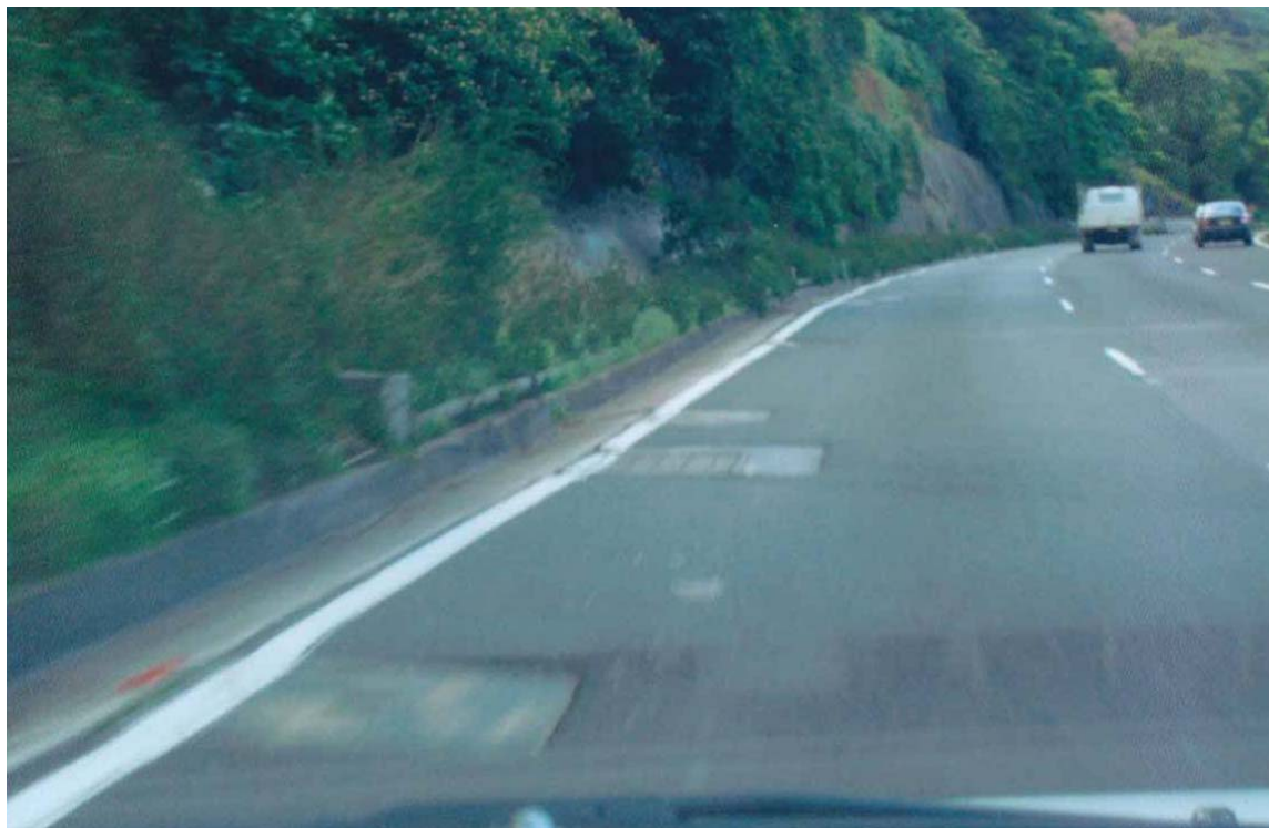
Note: Pit lids have settled causing deep ruts
