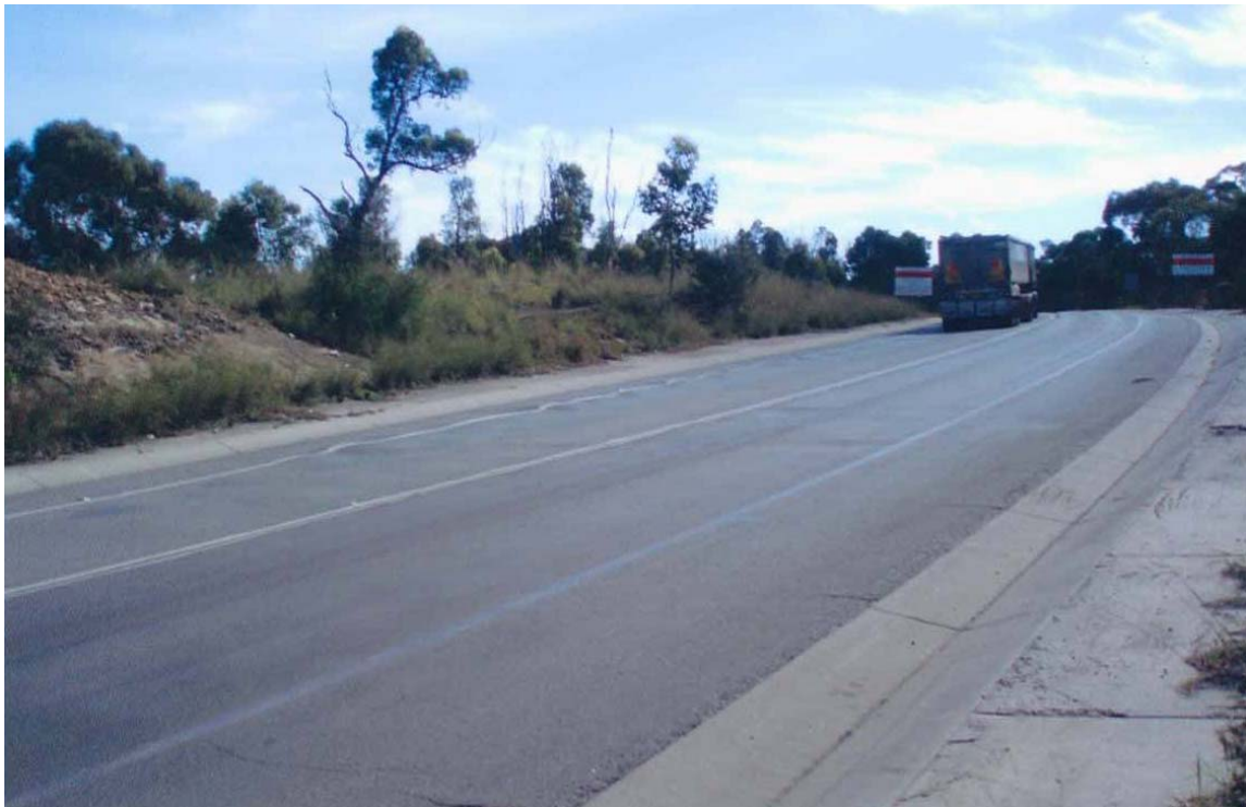
Photograph 3.7 View along access road showing heavy rutting along LHS pavement
