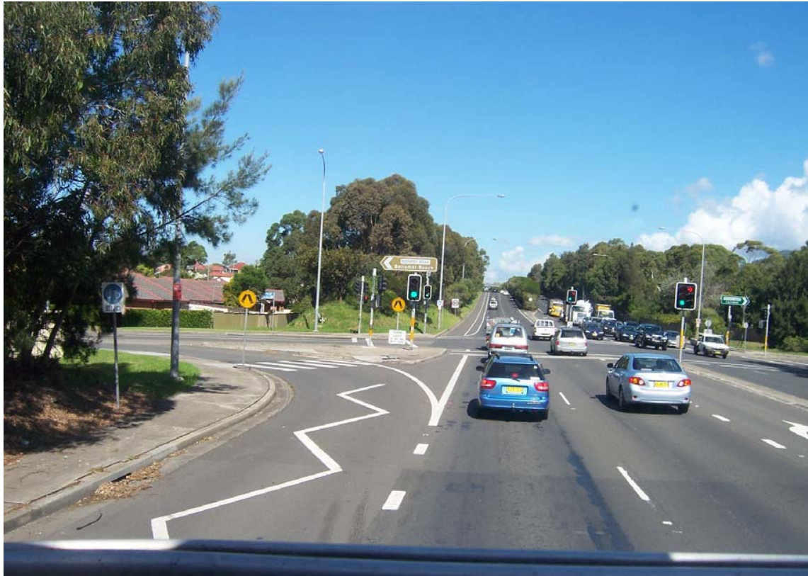
Photograph 3.17 Intersection of Northern Distributor and Towradgi Road
