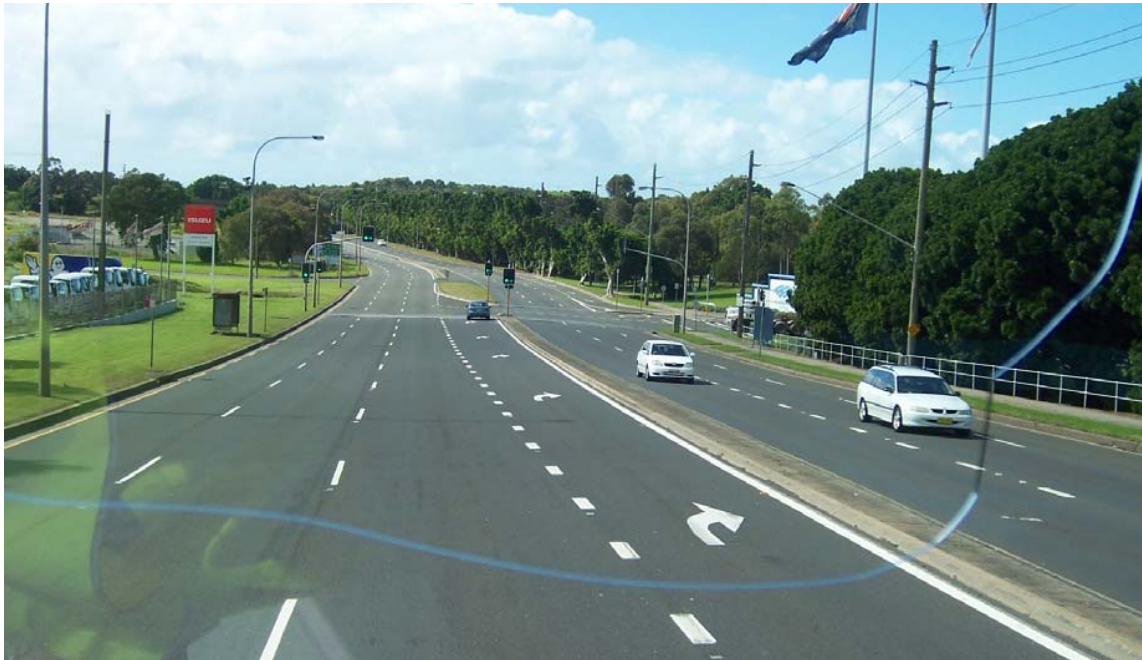
Photograph 3.14 Masters Road showing typical cross section
