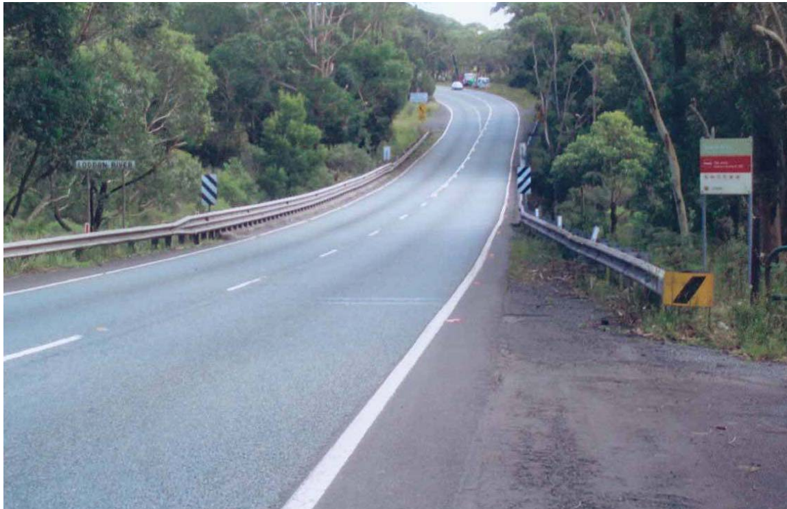
Photograph 3.8 Loddon River Bridge on Appin Road showing narrow width
