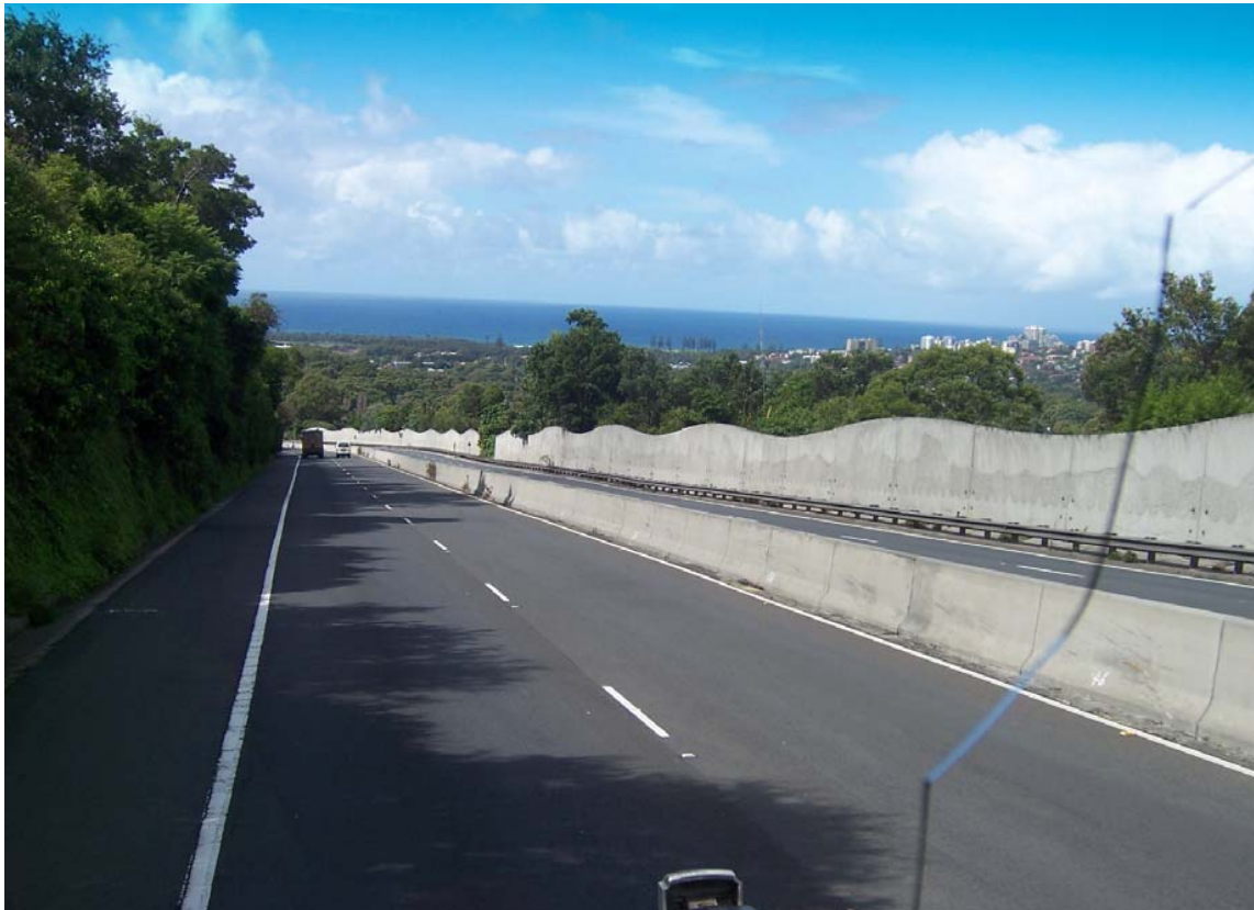
Photograph 3.12 Mt Ousley Road approaching the F6 freeway junction
