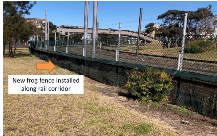
Figure 34 : Shade-cloth GGBF exclusion barrier along rail corridor
