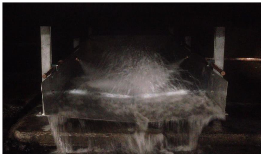
Figure 22: NC1 under-pan wash down system in action
