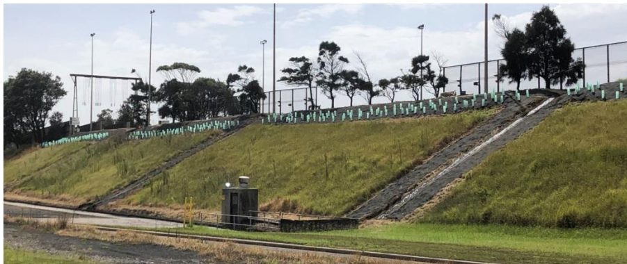
Figure 35 : Tree Planting - Northern Road Receival Berm (1)
