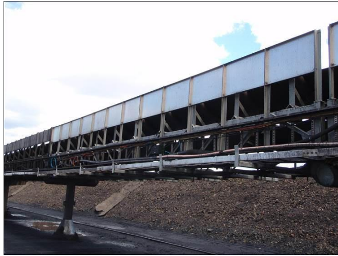
Figure 19: New Gantry and Windshields to improve dust control.
