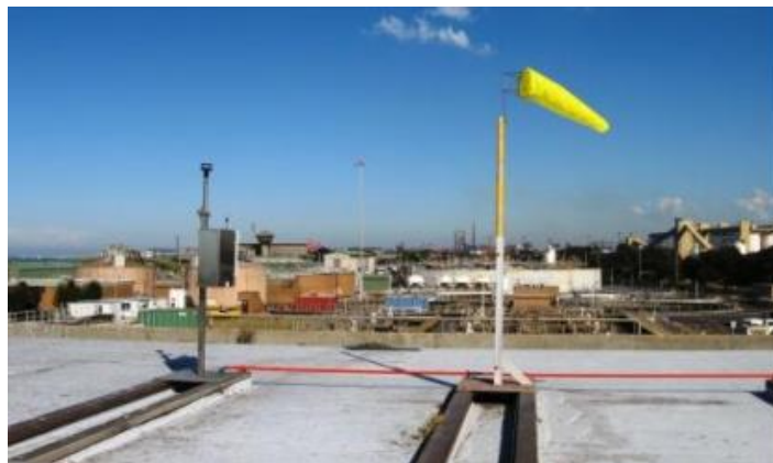
Figure 23 : PKCT northern continuous dust monitor
