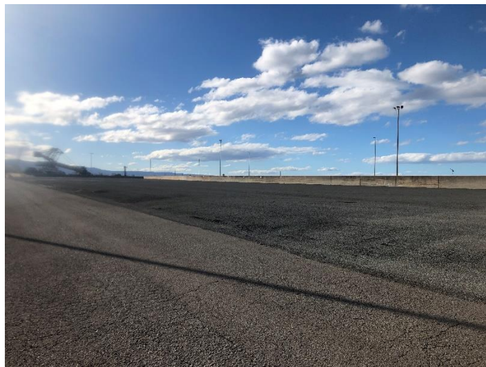
Figure 21: Completed Bulk Product Area Rectification and Resurfacing
