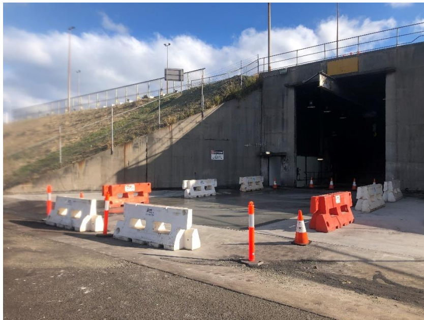
Figure 20: Newly sealed area near Road Receiving Station to limit dust generation
