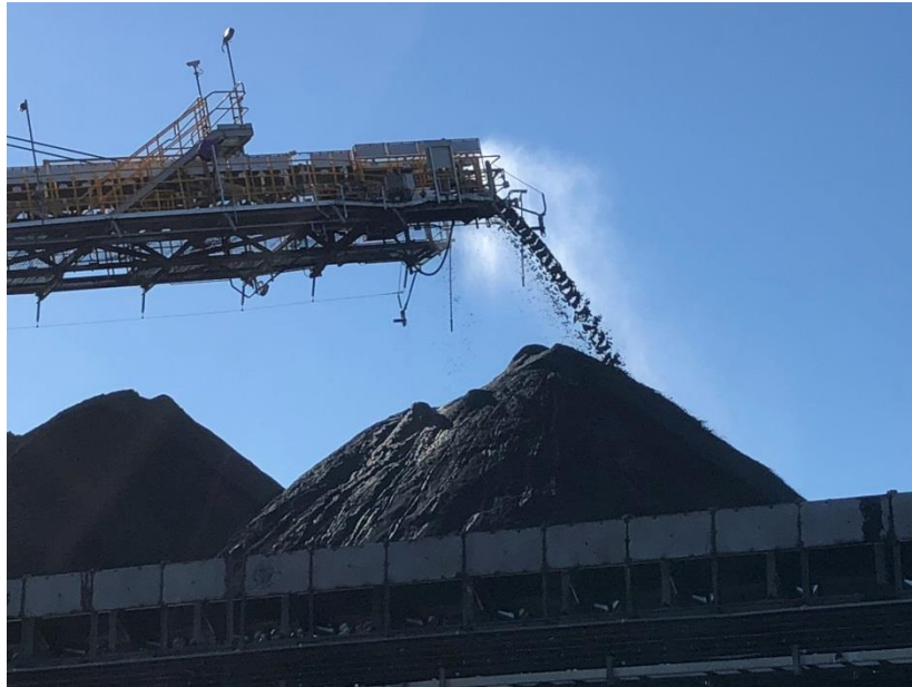
Figure 20: PKCT's new Stacker showing misting sprays during stacking to prevent dust
