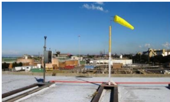
Figure 22: PKCT northern continuous dust monitor
