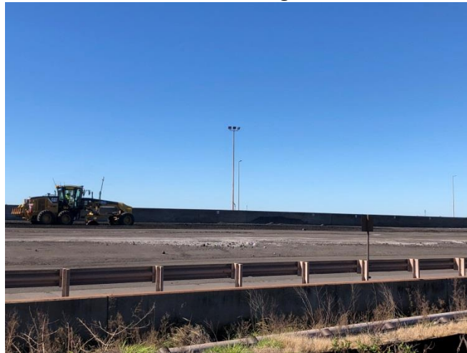
Figure 19: Progress of Bulk Product Area Rectification and Resurfacing
