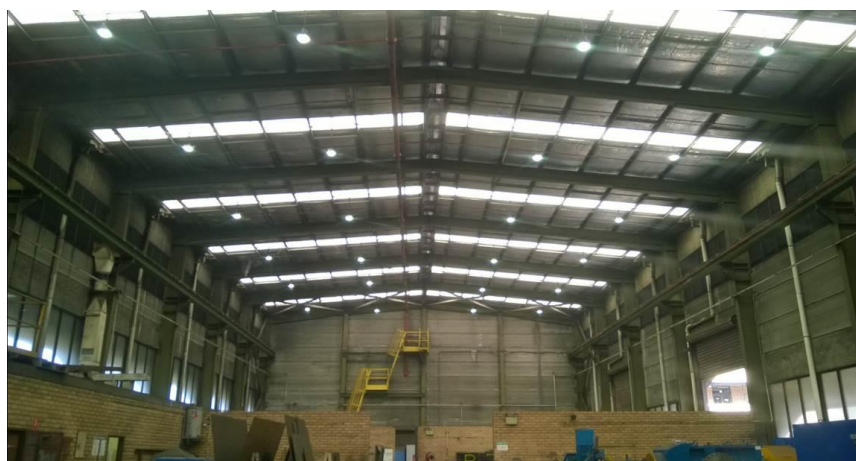
Figure 38: New LED lighting shown in the roof of the PKCT workshop
