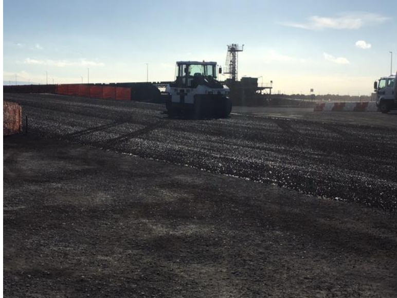
Figure 20: Bitumen sealing of southern access road
