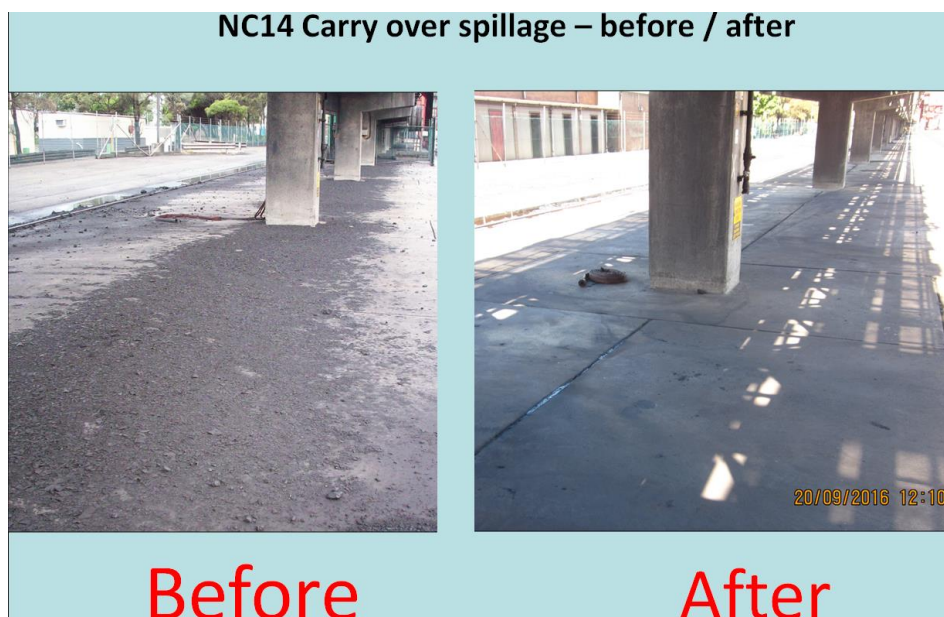
Figure 19: NC14 Belt scraper project before and after images
