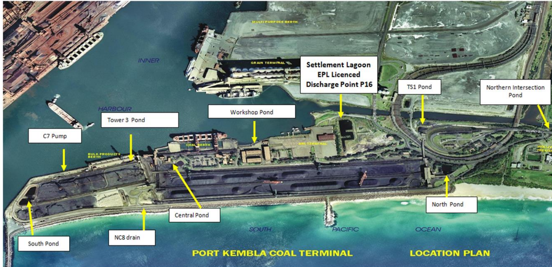
Water Collection System- Aerial View
