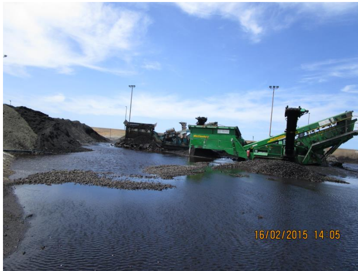
Figure 38: Ballast screening plant during rail upgrade project.
