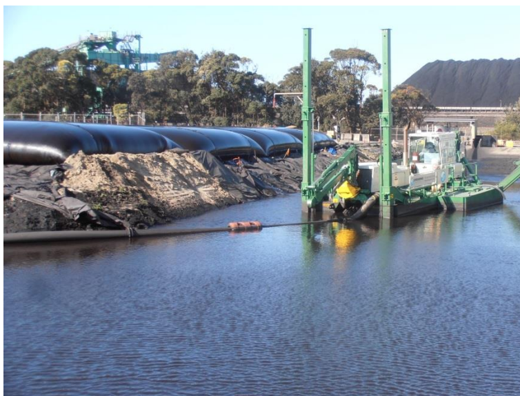
Figure 25: Dredging of Settlement Lagoon
