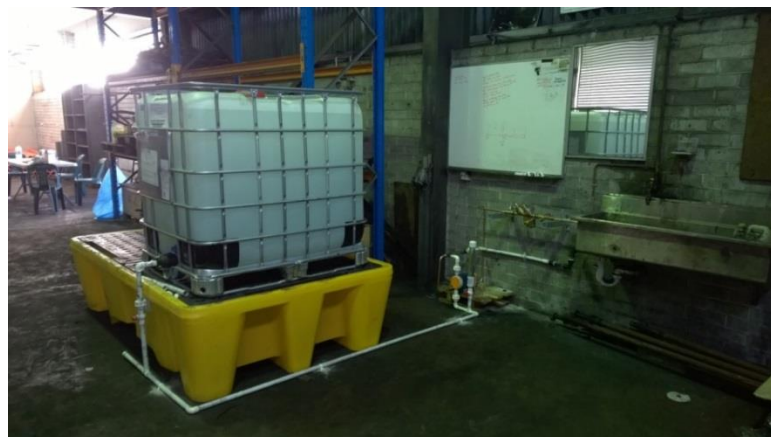
Figure 24: Coagulant dosing system installed at the Central Pond to assist with clarification of water entering the Settling Lagoon.
