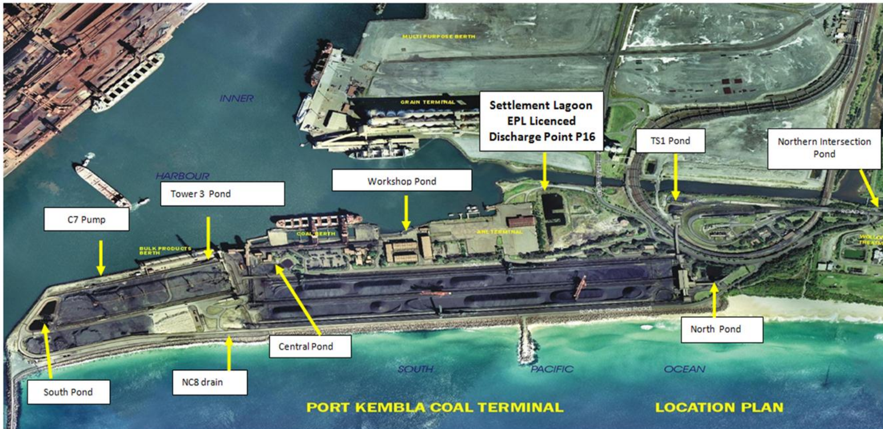
Water Collection System- Aerial View
