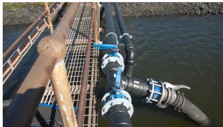
Figure 25: New pipework installed at LDP16 in the Lagoon to assist with controlled dewatering
