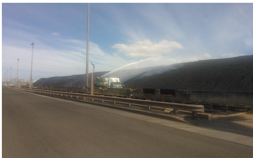
Figure 17: New fencing around Dust Gauge P4 to prevent vandalism of gauge and veneering of southern stockpile
