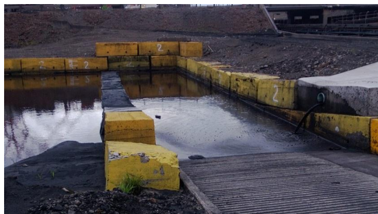
Figure 26: Installation of concrete blocks in Central Pond
