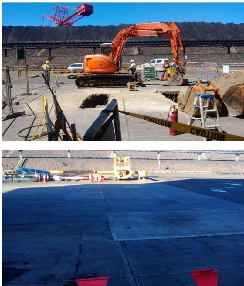
Figure 40: Decommissioning of underground fuel storage tanks
