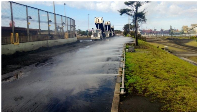
Figure 17: Road Receptacle dust suppression sprays
