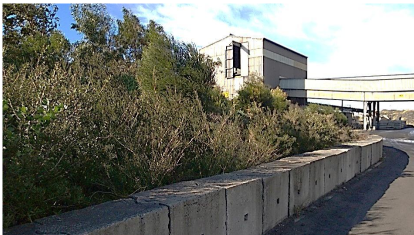
Figure 30: Landscaped area near Northern Transfer Station
