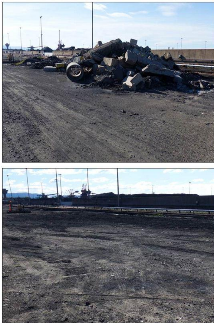
Figure 38: Removal of concrete from laydown area near Berth 101
