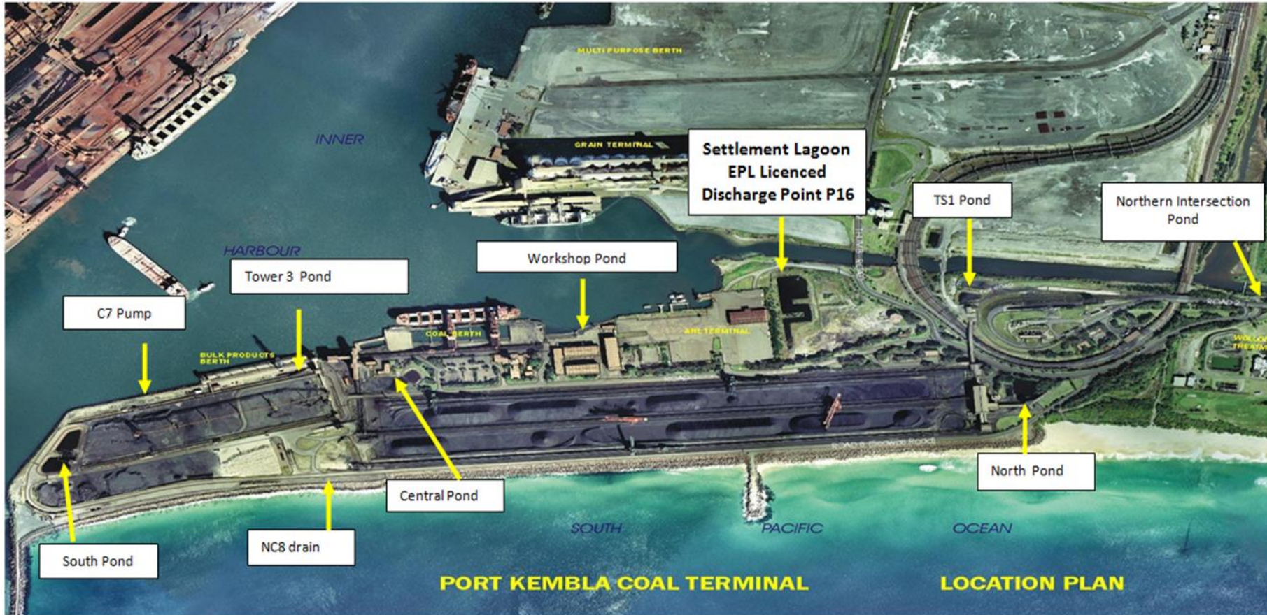
Water Collection System- Aerial View
