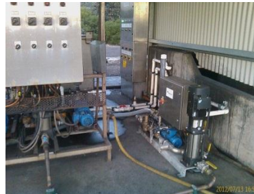
Back up dosing unit
