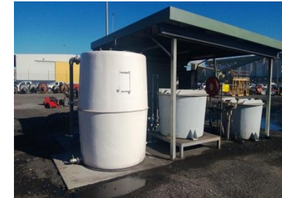
New polymer storage tank
