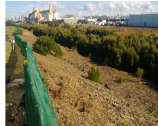
Improvement works adjacent to Garungaty Waterway
