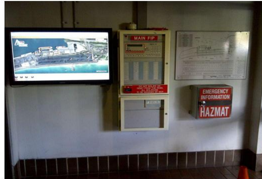
NSW FIRE BRIGADE- Display screen, fire panel, site plan
