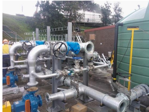
New spray pumps at the north truck wash
