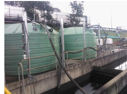
New water treatment facilities including sand filters
